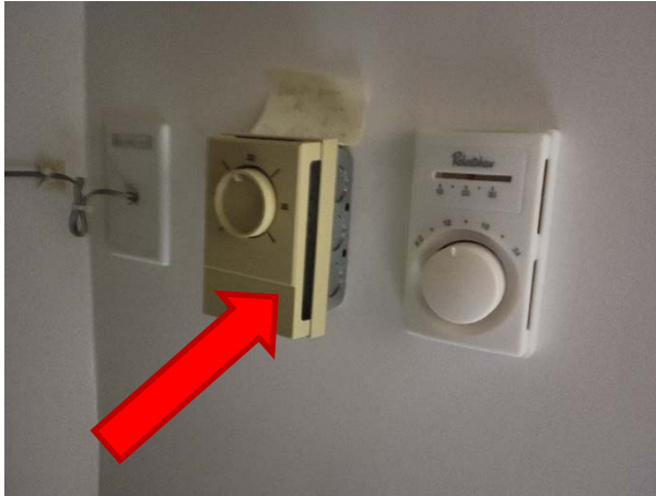
Thermostats could not be dismantled and should be inspected for mercury prior to disposal.
