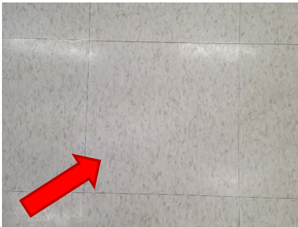
Beige with brown flecks 12" vinyl floor tile and mastic does not contain asbestos (S-006A-C).
