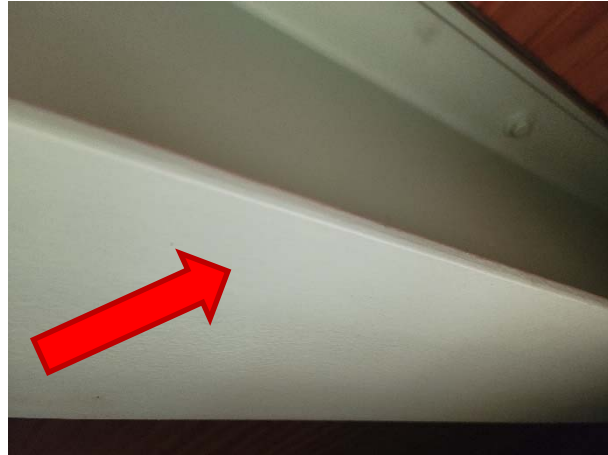
Green primer on structural steel contains elevated concentration of 0.1350% lead (LP04).
