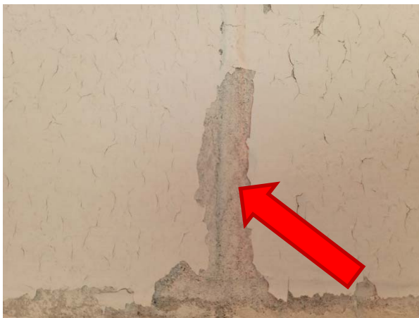
Concrete mortar found throughout the site in the concrete block walls does not contain asbestos (S-014A-C).
