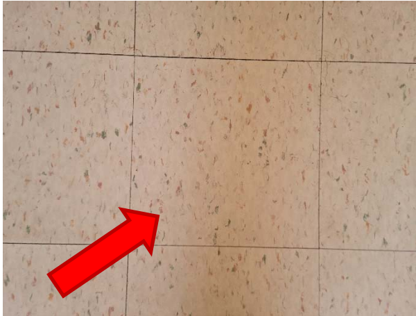
Orange and green flecks 12" vinyl floor tile and mastic does not contain asbestos (S-008A-C).
