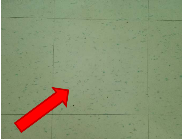
Light blue 12" vinyl floor tile and mastic (S-002A-C) does not contain asbestos.
