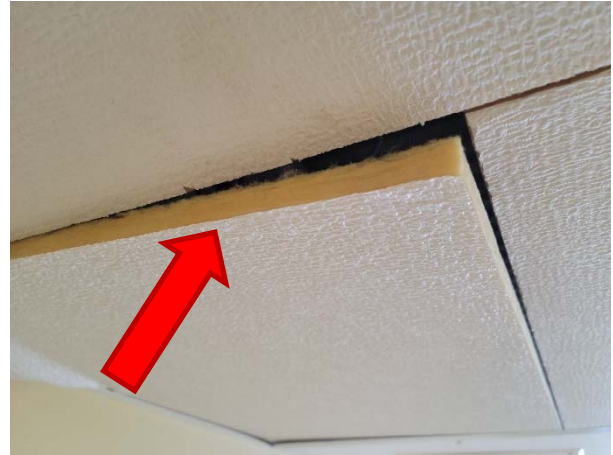
24" x 48" white fiberglass acoustic ceiling tiles are known not to contain asbestos.
