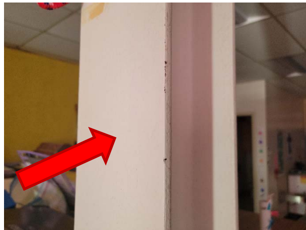
Beige primer on structural steel contains 0.0526% lead (LP06).
