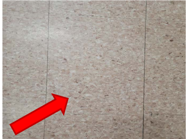
Pink and white 12" vinyl floor tile and mastic does not contain asbestos (S-009A-C).
