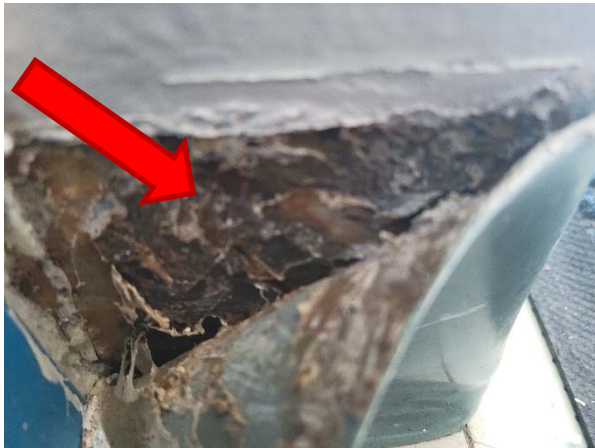
Brown mastic on blue vinyl baseboards does not contain asbestos (S-003A-C).
