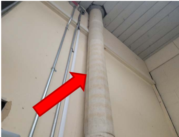
Canvas wrapped pipe insulation does not contain asbestos (S-011A-C).
