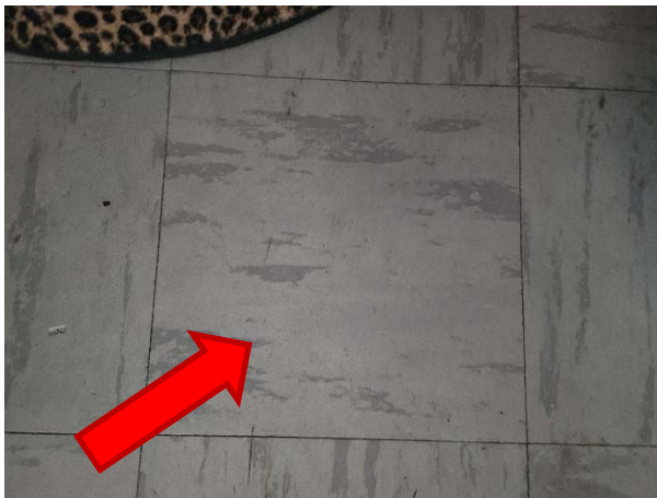
Grey 9" vinyl floor tile and mastic contains chrysotile asbestos (S-012A-C).
