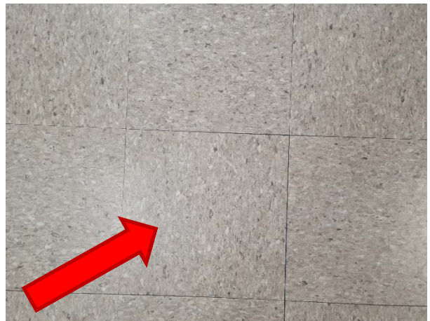
Black and brown flecks 12" vinyl floor tile and mastic does not contain asbestos (S-007A-C).
