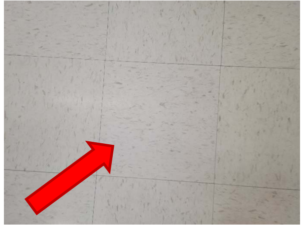
White with brown flecks 12" vinyl floor tile and mastic (S- 005A-C) does not contain asbestos.
