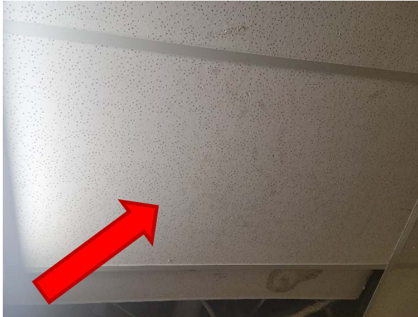
24" x 48" white with pinholes acoustic ceiling tile does not contain asbestos (S-001A-C).
