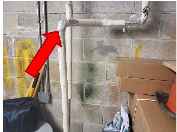
Foil wrapped fiberglass pipe insulation is known not to contain asbestos.
