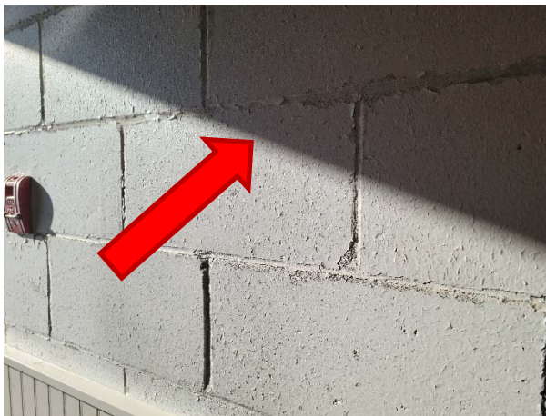
White paint on concrete block contains 0.0018% lead (LP05).
