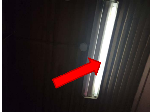
Mercury vapour is present in florescent lamps. Ballasts should be inspected for PCB prior to removal.
