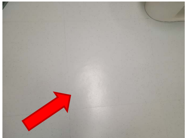
Light grey 24" vinyl floor tiles are known to not contain asbestos based on size and estimated age.
