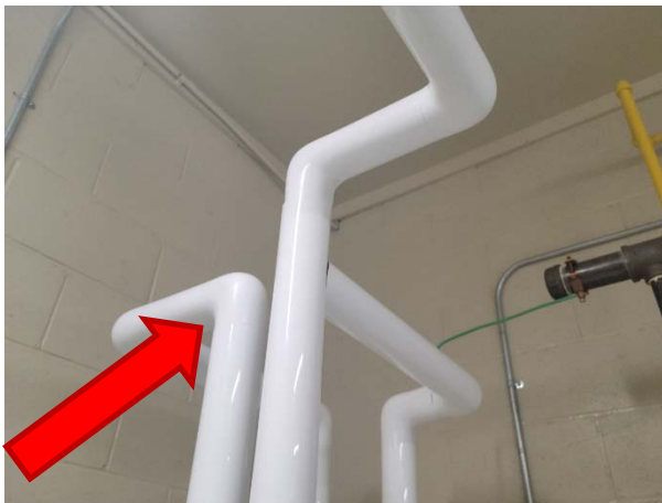
Plastic wrapped fiberglass pipe insulation is known not to contain asbestos.
