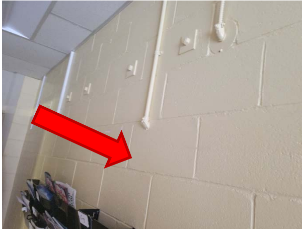
Yellow paint on concrete block contains 0.0116% lead (LP03).
