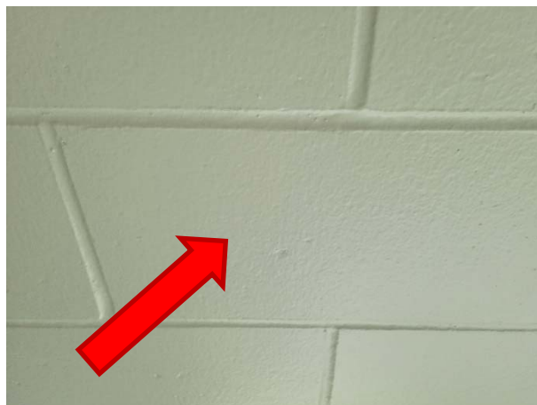
Beige paint on concrete block contains 0.0280% lead (LP01).
